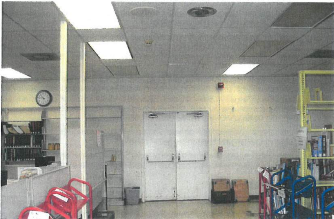
Photo 7. Unbraced Original 2' x 4' Suspended Ceiling Grids in Service Building
