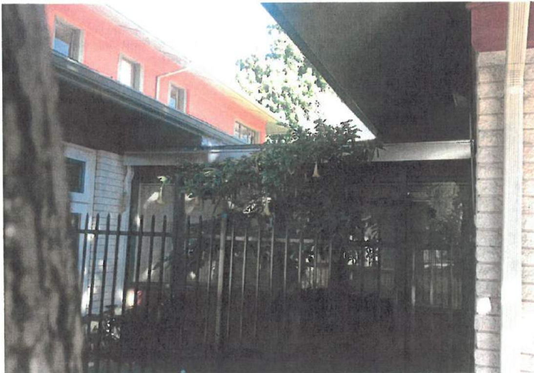
Photo 5. Connecting Link between Main Building and Service Building
