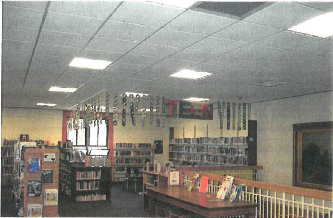
Photo 6. Braced Replacement 2' x 2' Suspended Ceiling Grids in Main Building
